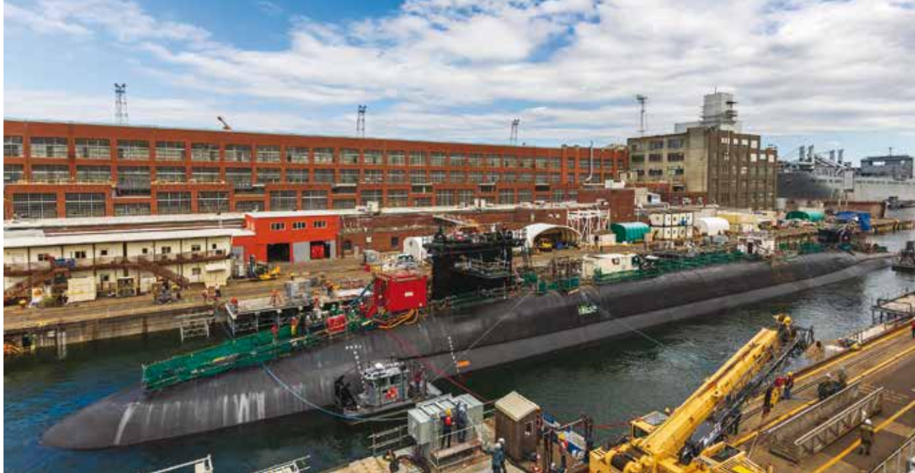
USS Maine (SSBN 741) in Dry Dock 4 at Puget Sound Naval Shipyard and Intermediate Maintenance Facility in Bremerton, Washington, June 2018.
