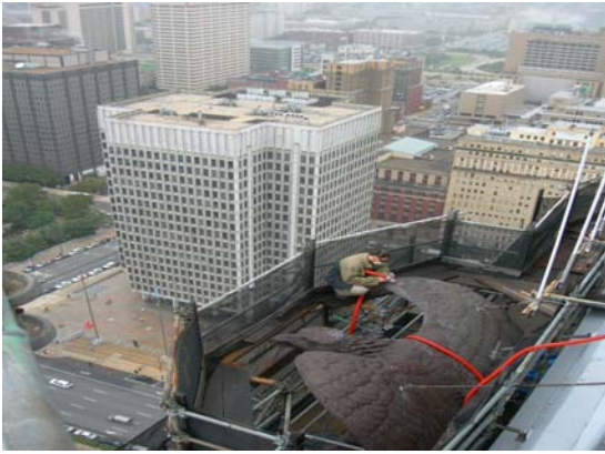
Figure 2. Fiber Optic Delivery
