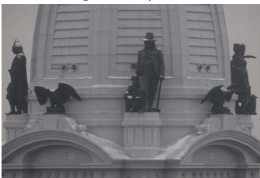
Figure 1. Philadelphia City Hall Tower Statue Corrosion Cleaning
