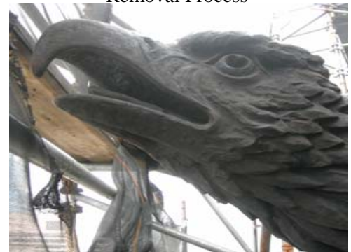
Figure 5. After Corrosion Removal Process
