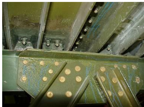
Figure 2: Fuel tank topcoat blistering in a P-3 aircraft (FRC-SE)
