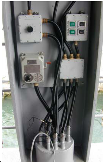
Figure 7 – New Composite Electrical Enclosure Installation for Stern Gate Controller
