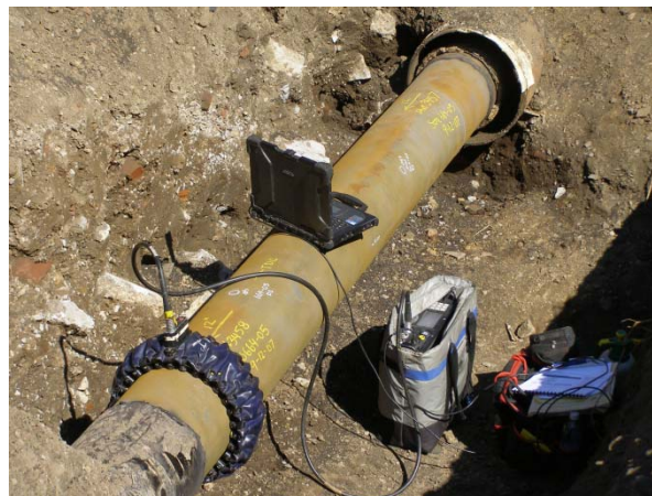
Figure 1: GWUT equipment setup in an excavation.
