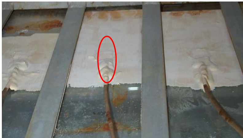
FIGURE 8. Test panels consisting of water-borne epoxy coating painted over LPR sensors.
