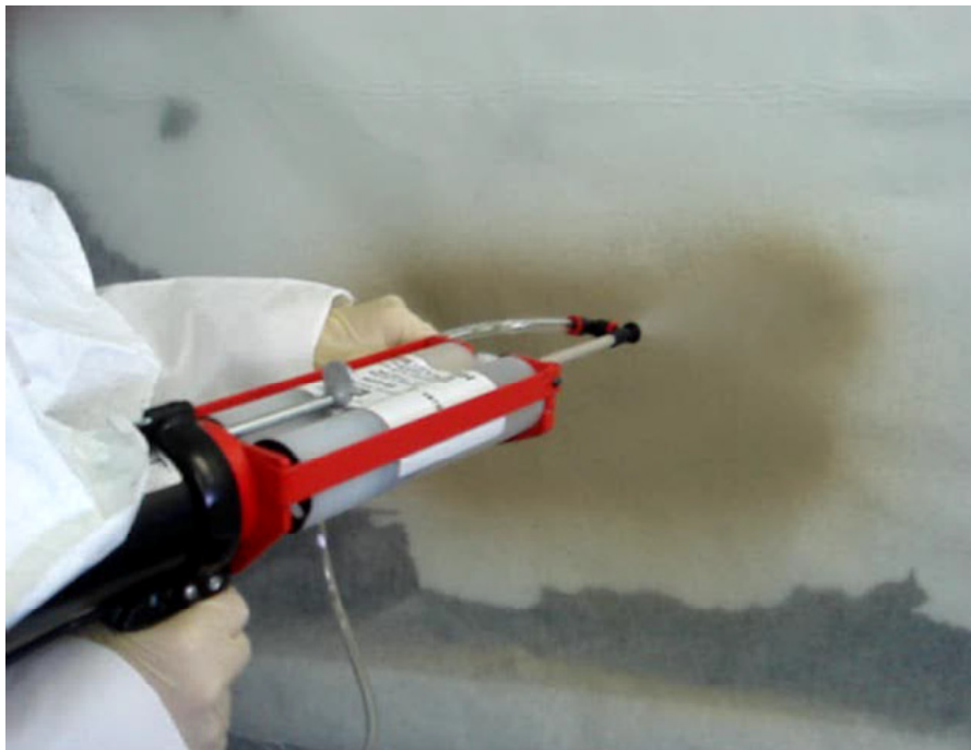
Figure 2 – Example of Polyurea Coating Cartridge Spray Application.
